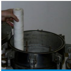
5. Install new filter cartridges
