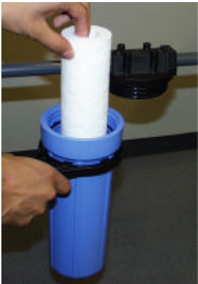
2. Exchange filter element
